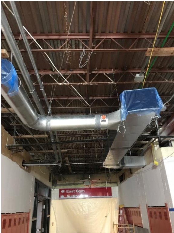
Installed Duct Work
