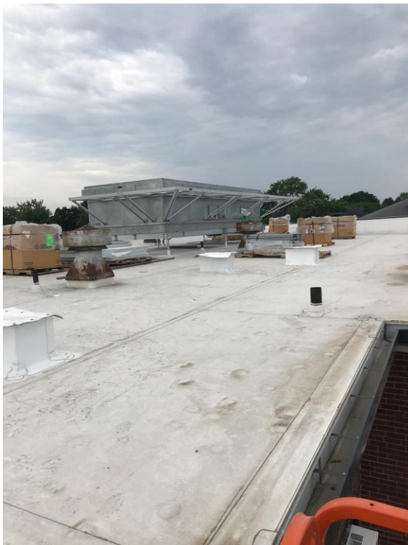
Installed RTU Curb Catwalk
