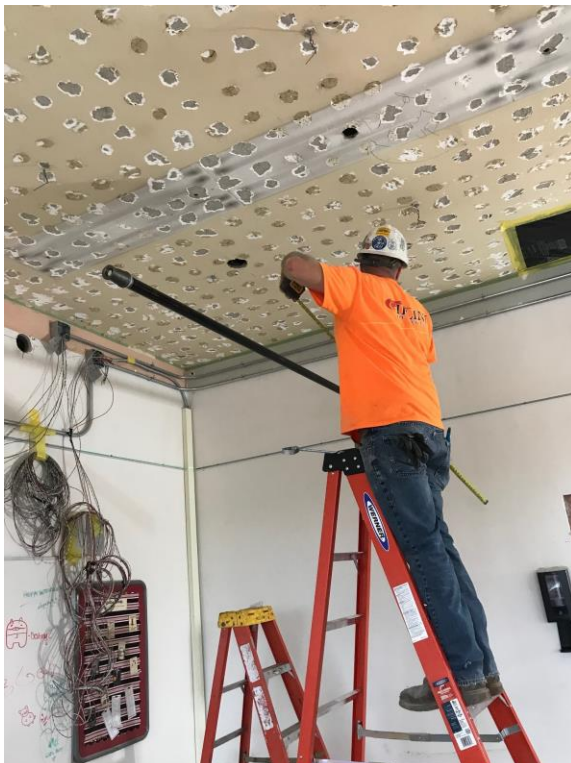
Sprinkler Pipe Installation
